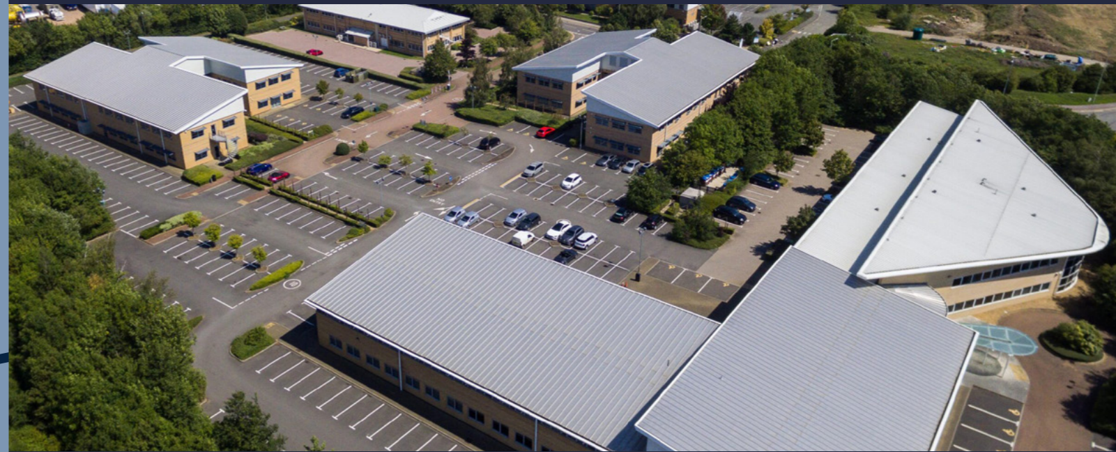
Aerial view of Cranfield University Technology Park
